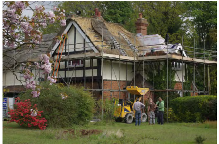
"Work to remove the thatch on the last thatched estate house in the village begins"
